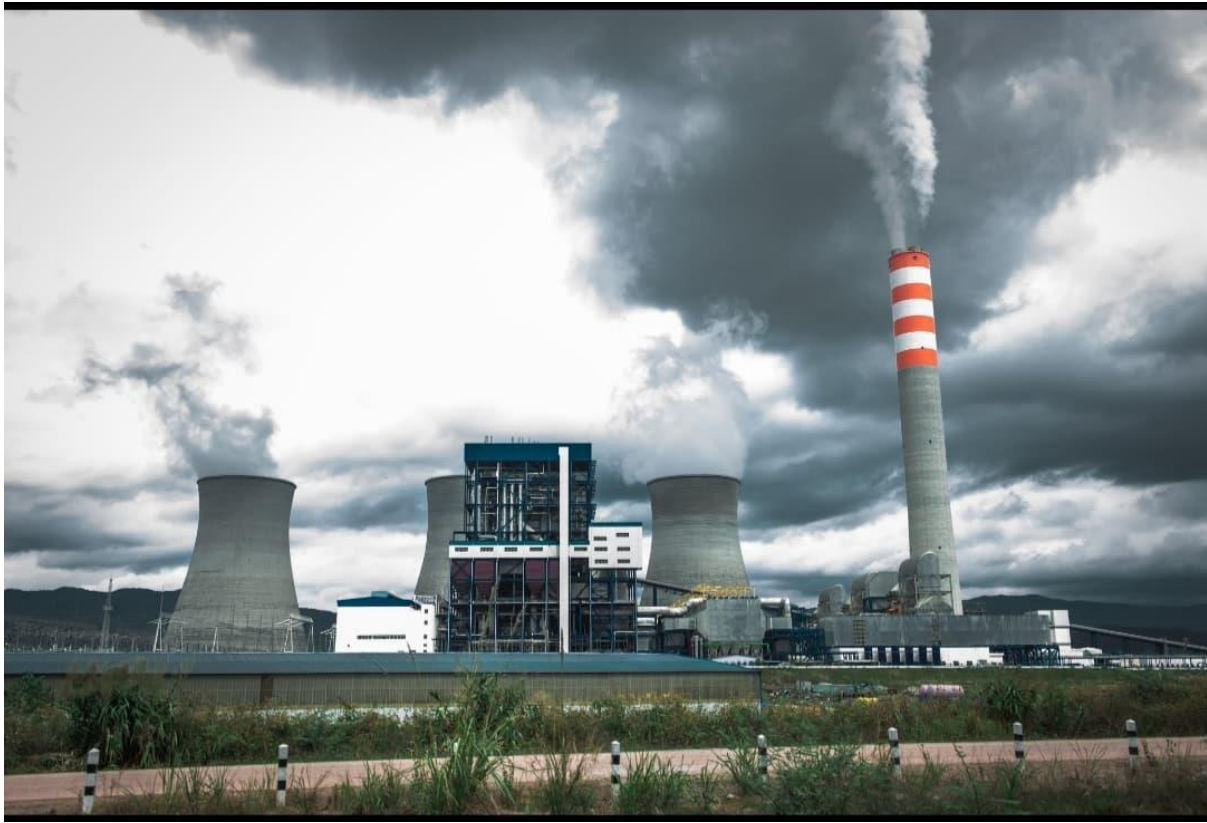
Hongsa Lignite Power Plant Project Area: photo by Jamon Sornpetchnarin
